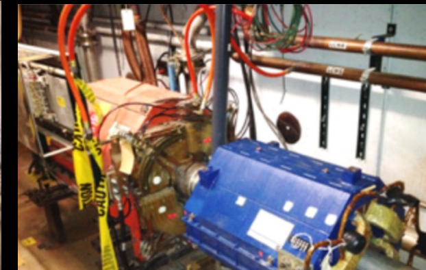
Quadrupole in Delivery Ring used for resonant extraction
